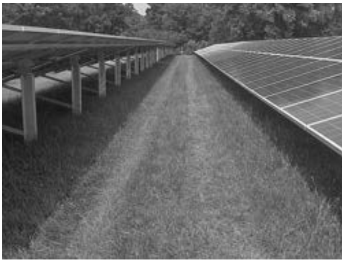
Fig. 1. Maintenance or “spacer” section between two rows of solar panels (photo by John E. Showler, reprinted with permission)
