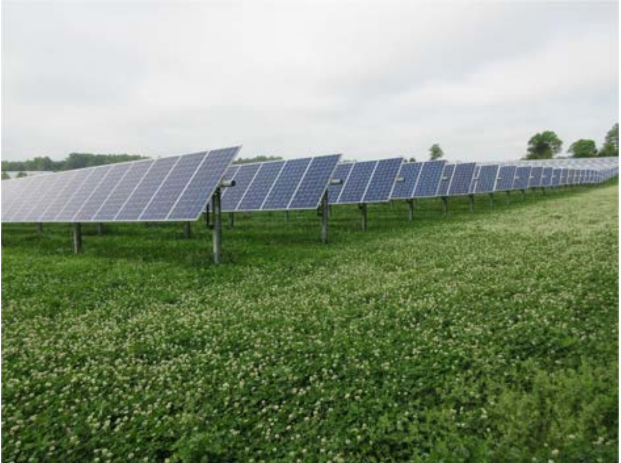
Figure 2. Typical Single-Axis Tracker System
