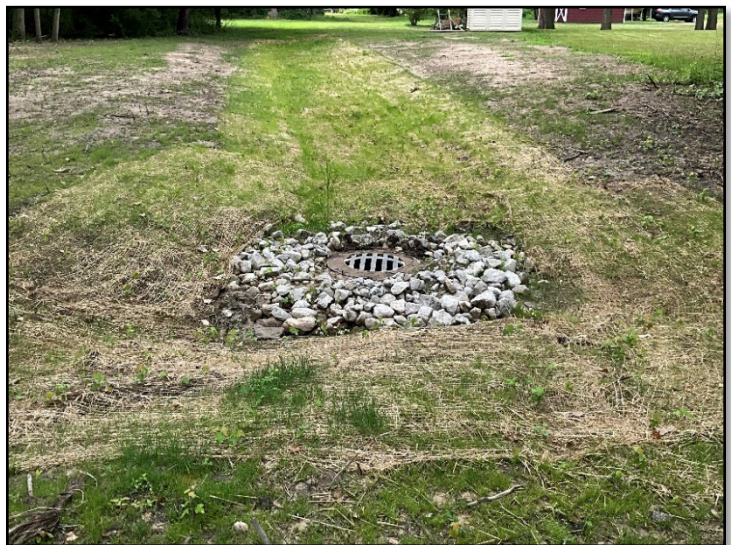
Installation of a new branch drain with underground pipe and catch basin surface inlets.
