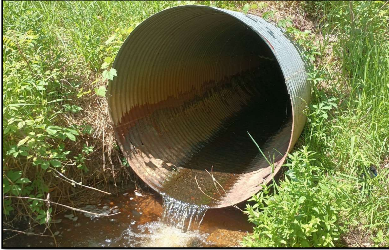
Failing Road Culvert, 48 th Avenue, Covert Township (County Line Road)
